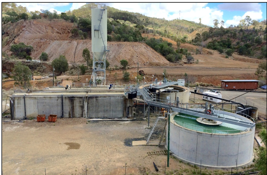
Figure 1: The Mount Morgan water treatment plant
